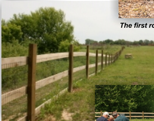
Finished section- May 17th
